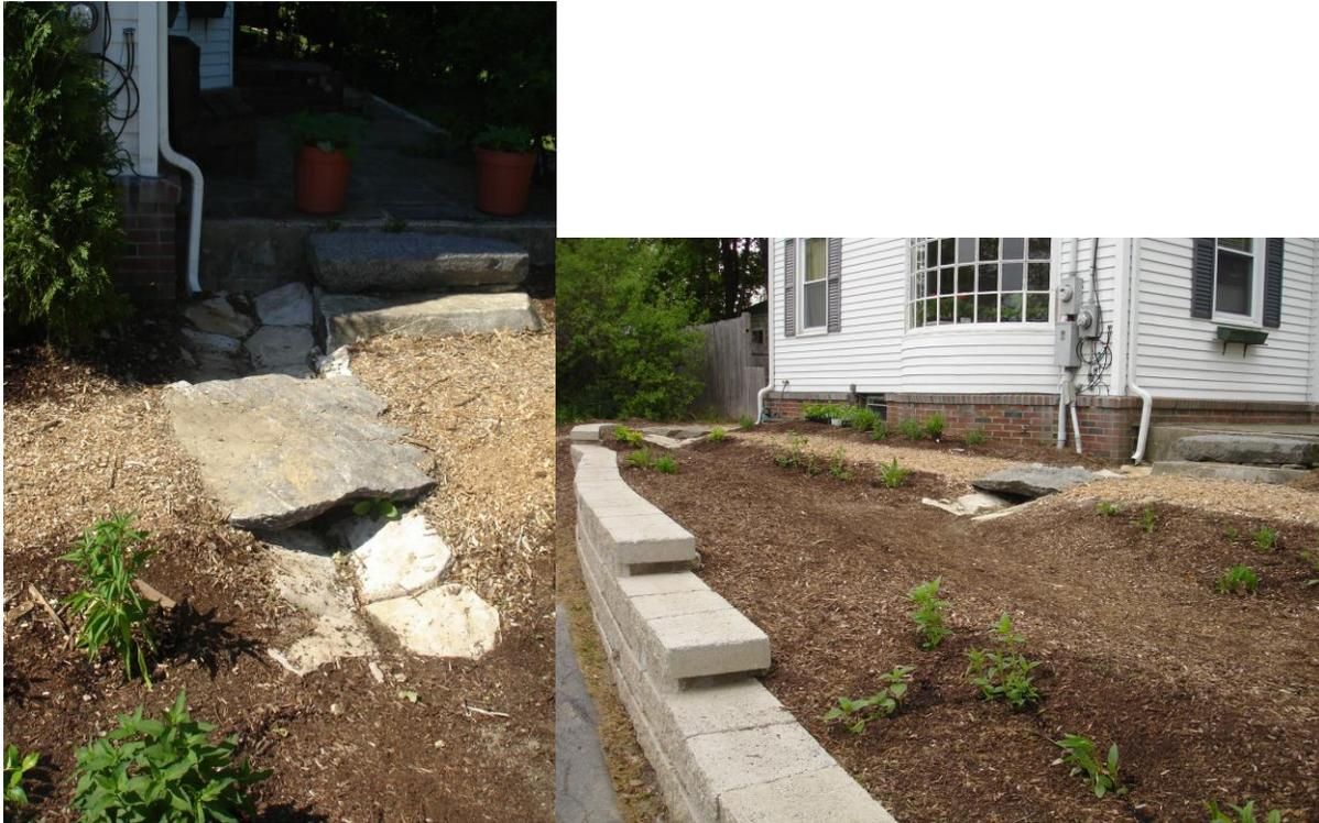
Construction photos show how gutter downspouts dump to a stone-lined channel then through a mulched swale to a depressed planting bed.
