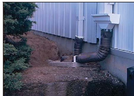
By redirecting a drain spout from the parking lot to a vegetated area, Lampin Corporation of Uxbridge diverted more than 73,000 gallons of stormwater runoff per year.
